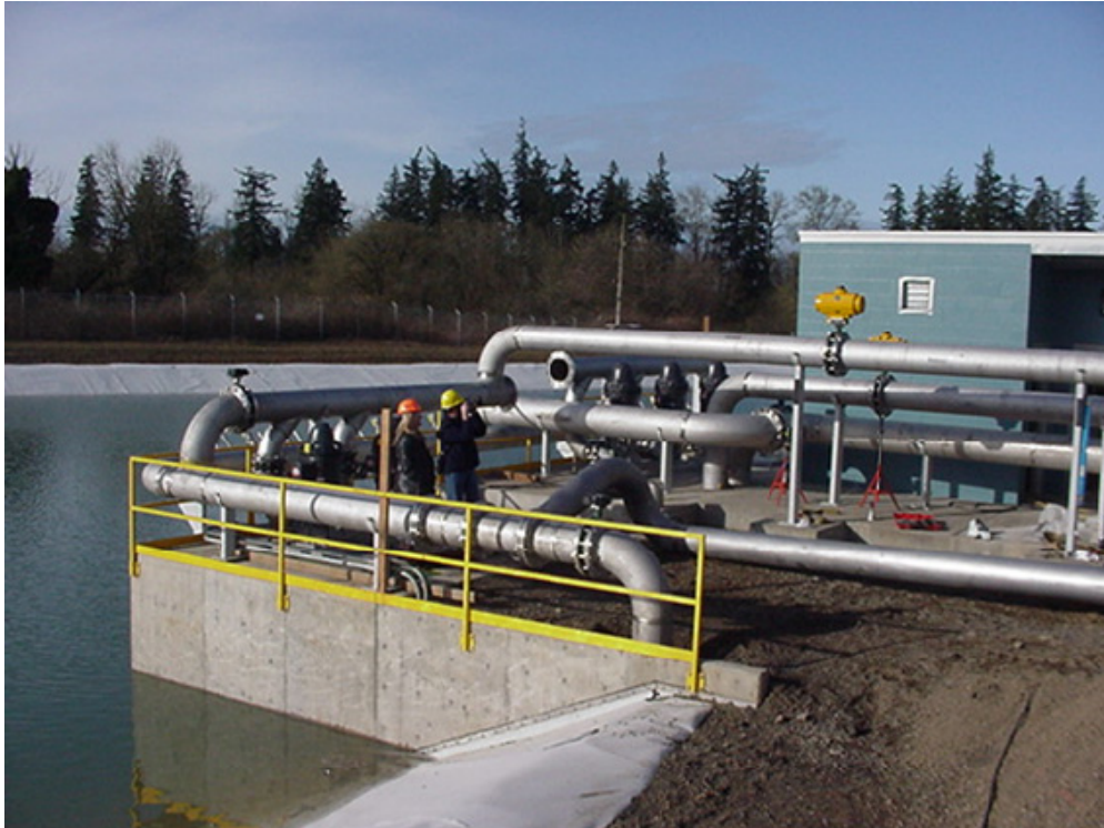
Figure 6: ATI 2102® pipes as installed at the pumping station.
