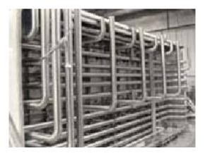
Figure 6: In-Plant Piping of UNS S20153 alloy
