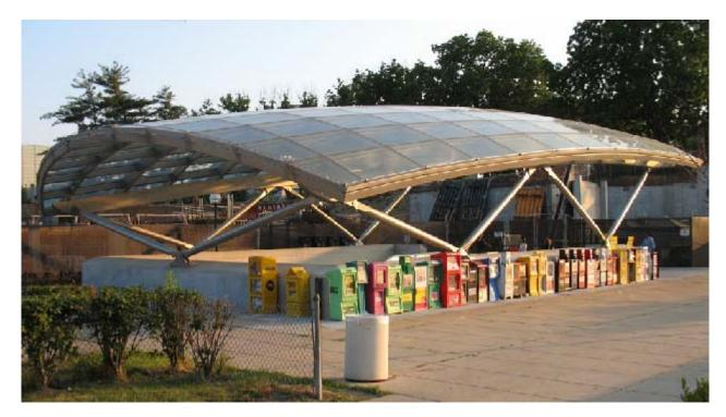
Figure 8: UNS S32003 alloy used in piping for structure support. Canopy from the Medical Center Metro Station in Bethesda, MD.
